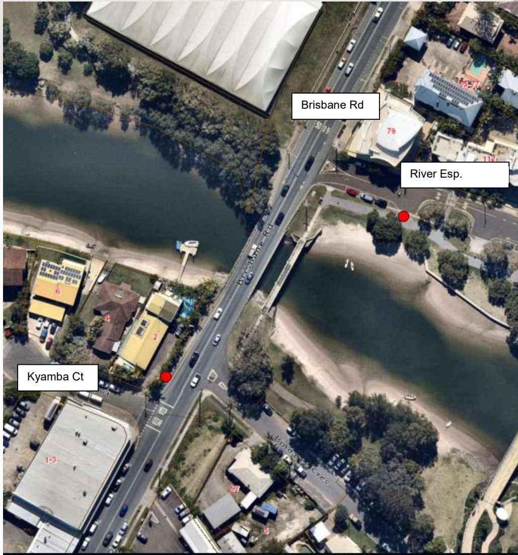
Figure 1 Location of potholing works Brisbane Road.
